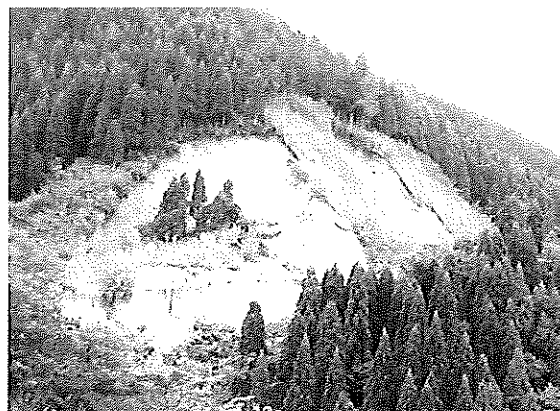
Photo 9 Collapse in road cut slope A
